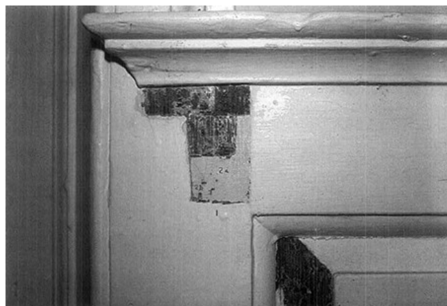
The paint chronology of this mantel, seen in the exposed paint layers in the left corner, proved it had been relocated from another room of the house. To remove a significant feature's paint history and the evidence of its original sequence of color by stripping off all the paint is inappropriate - and unnecessary - as part of a lead hazard reduction project. Careful surface preparation and repainting with lead-free top coats is recommended. Photo: NPS Files.
