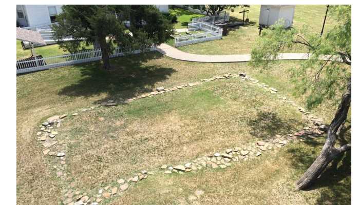
— Image above shows the original foundation outline still visible behind the main house
